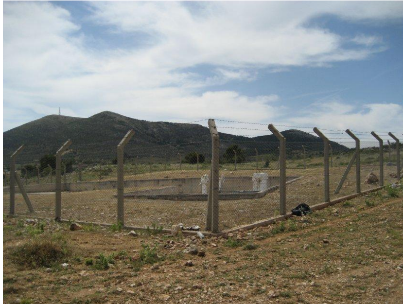
Fig 15. Valve station. Indicative Photo.
